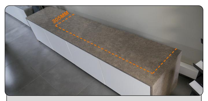
Check the width of the model you are installing below by scanning the QR code, and use a depth of <u>305mm</u>. Your cut-out depth will now line up with the top section of the unit, giving you approximately a 30mm overhang from the unit.
